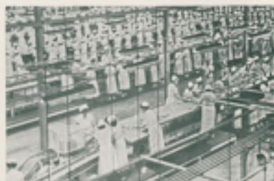
On spotter production line, fish are bled and filleted in preparation for canning.
